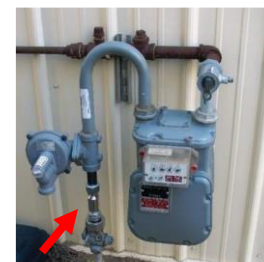
Figure 2 - Breakaway Fitting Provided By GTI
